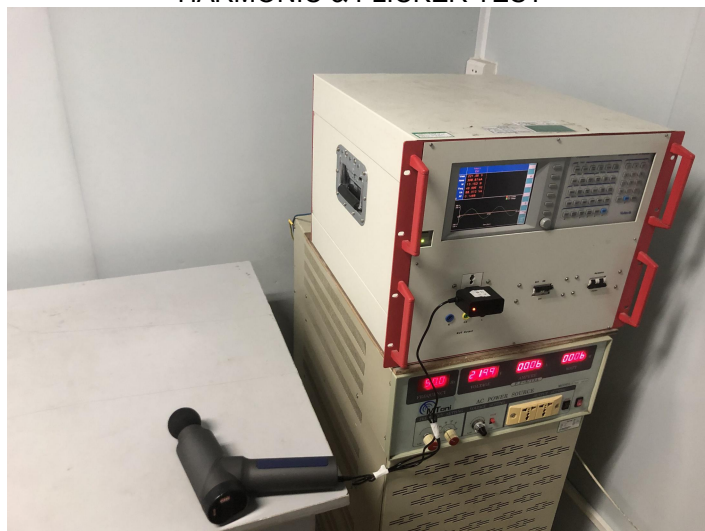
HARMONIC & FLICKER TEST
